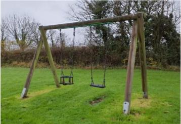
**Finding:** The inspector has some concerns about the internal condition of the timber cross bar (timber discolouration may indicate internal rot) and was unable to verify the structural integrity without further testing. We recommend a Resi-PD survey to establish the condition of the timber at it's core.
