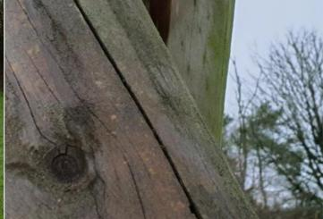
Finding: The timber elements have a number of splits/shakes or air cracks and this may affect the stability or fixing points of the structure and/or cause any instability allow water ingress which will accelerate the rotting process
